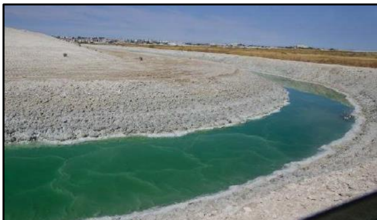
Figure 2: Leachate from the perimeter channel.
